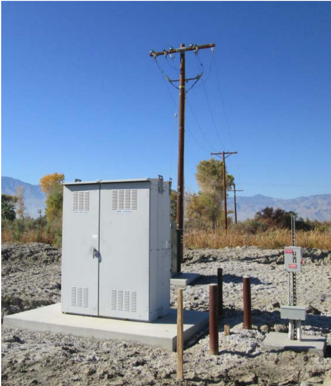
Existing Imperial Irrigation District Service (Pole and Main Service Panel)
